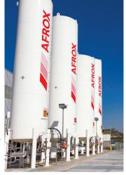
the event gas levels drop below pre-set levels. With this system, customers are able to monitor gas consumption as well as plan accordingly. Afrox is also able to use this data to re-fill the vessels based on set minimum levels
